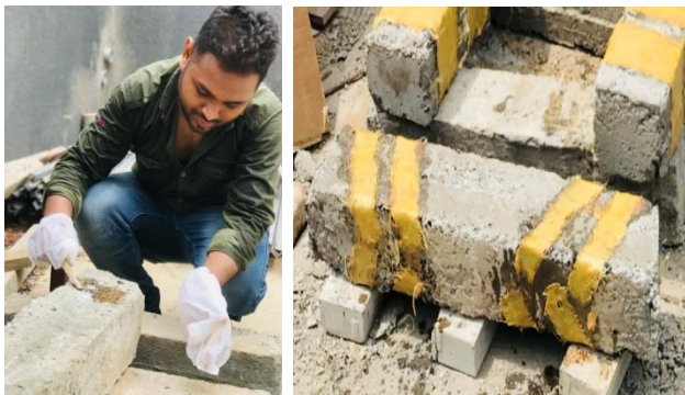
Fig 7 Applying resin and AFRP sheet 45° degree on beam M20 & M25
