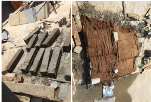
Fig. 2 De-Moulding and Curing
