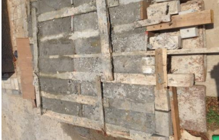
Fig 1 Casting of beam
