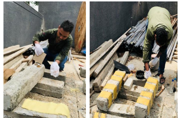
Fig 8 Applying resin and AFRP sheet Vertical Strip on beam M20 & M25
